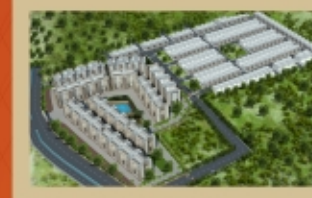
MAHALAXMIPURAM-PHASE-I BARAN ROAD, KOTA
