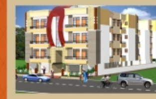
SURYA RESIDENCY, RAILWAY STATION, KOTA
